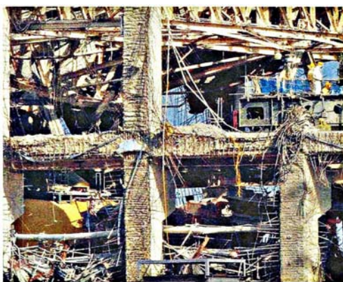
Fukushima Daiichi Reactor #4 after hydrogen explosion
